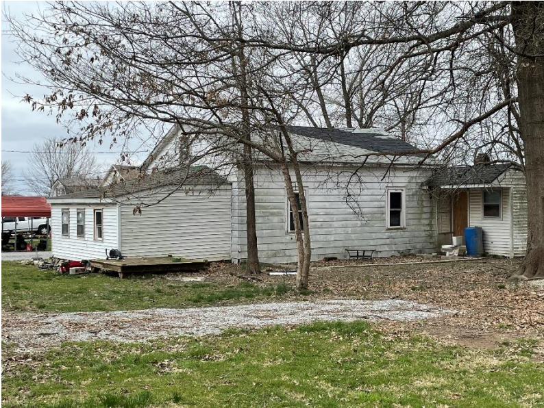
Figure 22. MN-740, side view, facing west.
