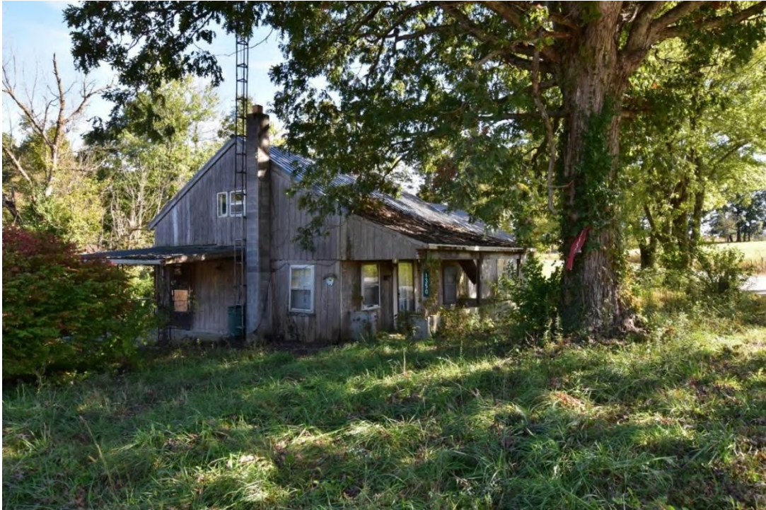
Figure 94. House says 1350, Google says 1240 Fairgrounds Road (37.557649, -85.230599).
