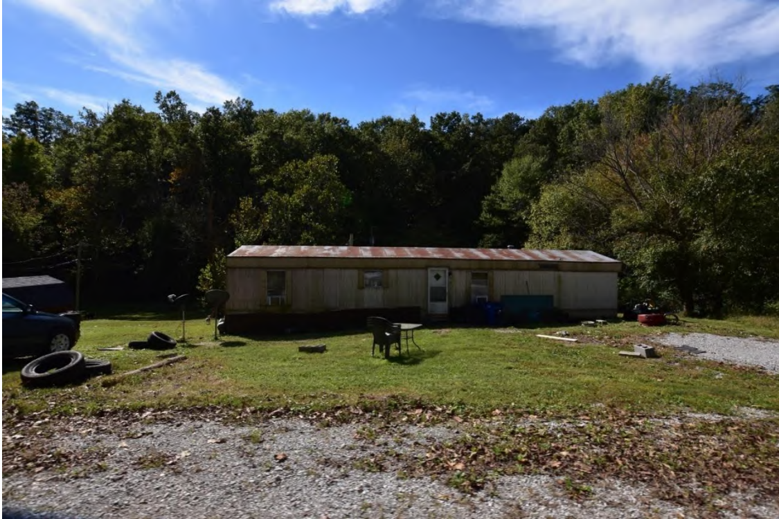
Figure 89. 1295 Sulphur Springs Road.
