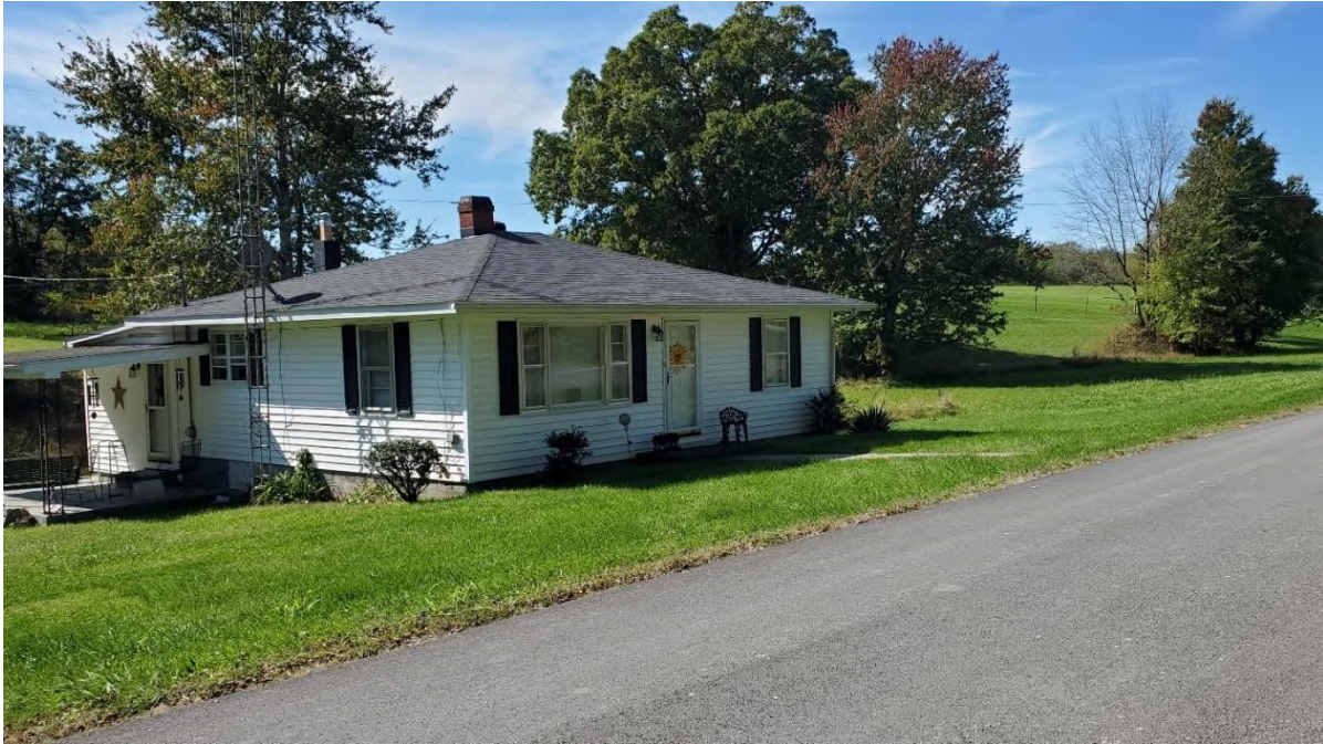
Figure 79. 875 Sulphur Springs Road.
