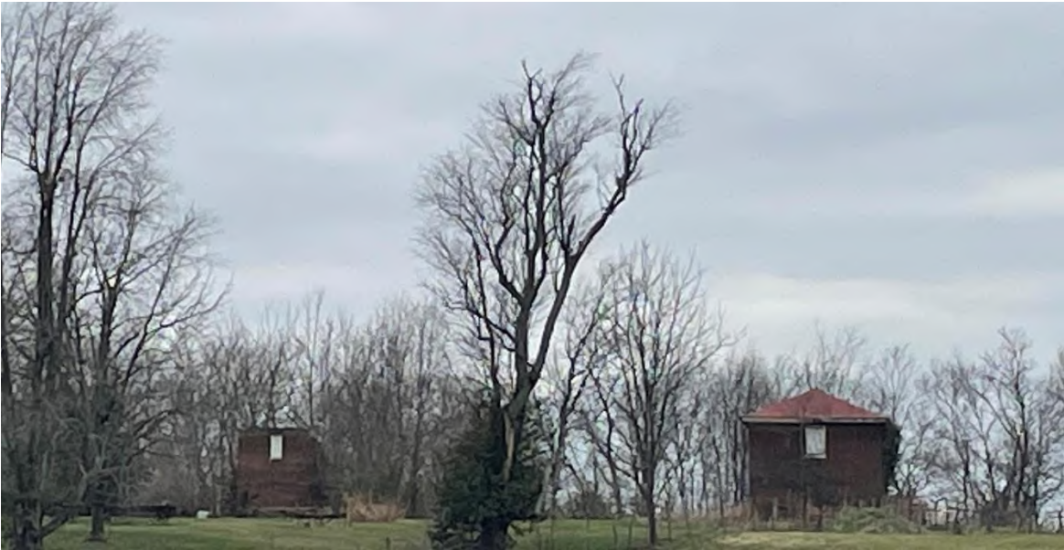
Figure 14. Outbuildings at MN-12.
