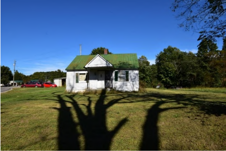
Figure 26. KHC Site Number MN-745. Fairground Road.
