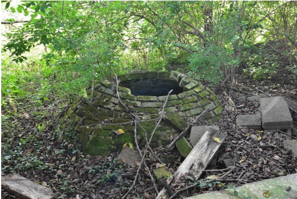
Figure 32. Cistern observed between the barn and associated silo at site MN-1104.
