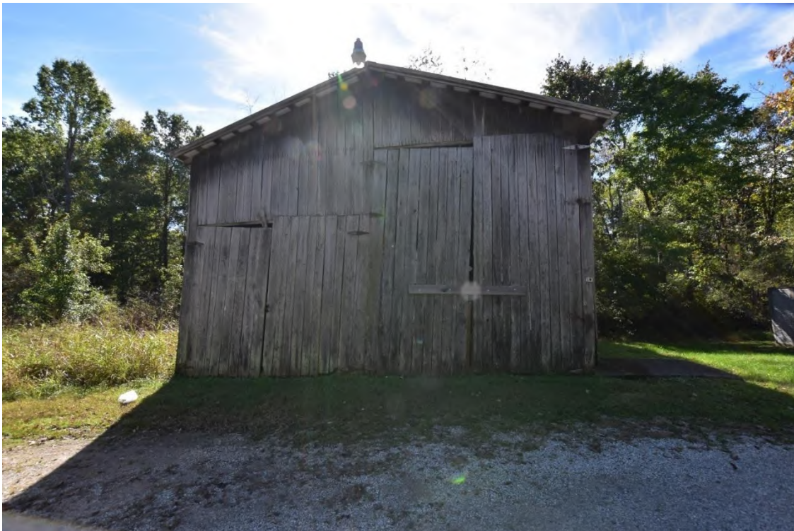
Figure 80. Barn in the yard of 875 Sulphur Springs Road.
