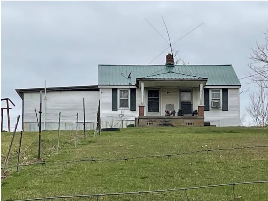
Figure 27. KHC Site Number MN-746, 1345 Fairground Road.
