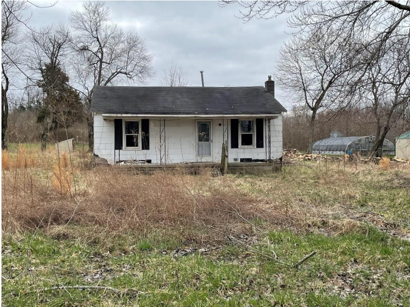
Figure 24. MN-742, 151 Hood Lane. Front view facing southeast.
