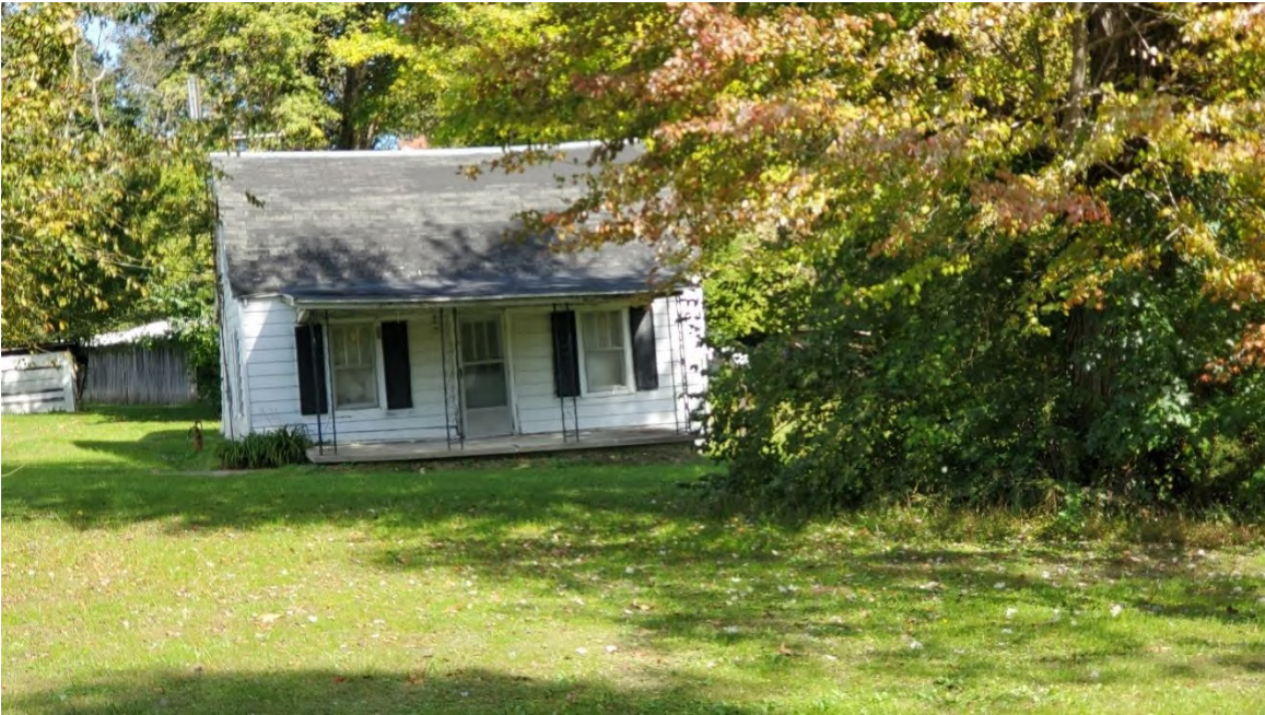
Figure 82. Sulphur Springs Road (37.565302, -85.221660).
