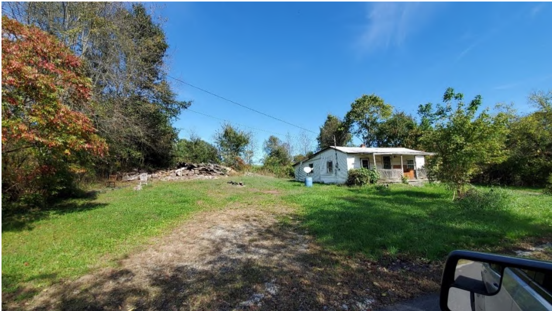
Figure 83. Sulphur Springs Road (37.565302, -85.222669).
