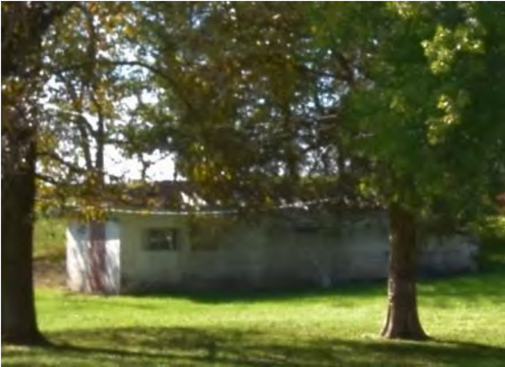
Figure 91. Structure or building in the backyard of 1031 Fairgrounds Road.
