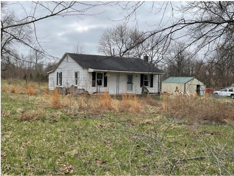
Figure 25. MN-742, 151 Hood Lane, side view facing south.
