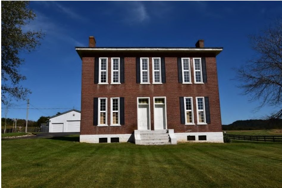
Figure 10. MN-10, 1670 Sulphur Springs Road.
