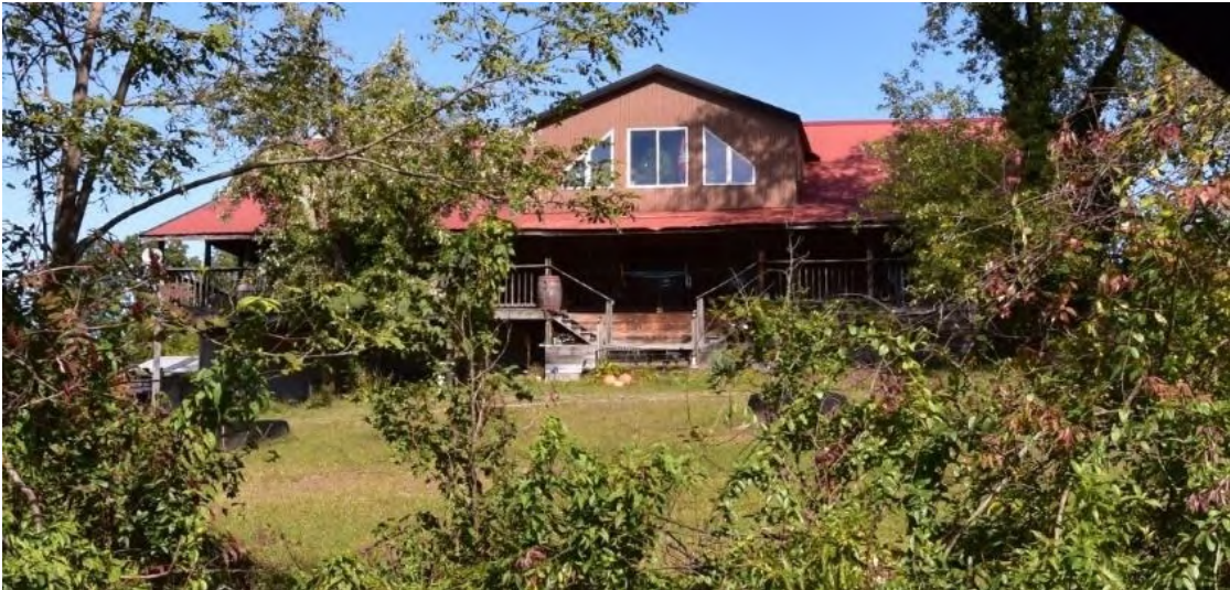
Figure 85. Sulphur Springs Road (37.566610, -85.223536).
