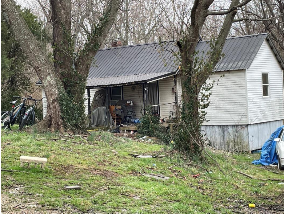
Figure 20. MN-738. 221 Hood Lane, side view, facing east.
